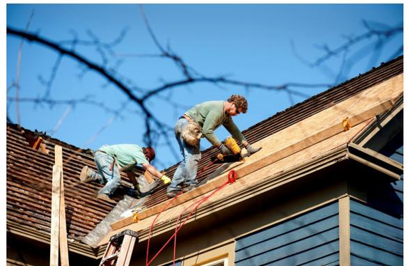
Workers building a roof. Sheets of plywood are covered by asphalt shingles, overlapping tiles, or other waterproof materials. Credit: Federal Emergency Management Agency.
