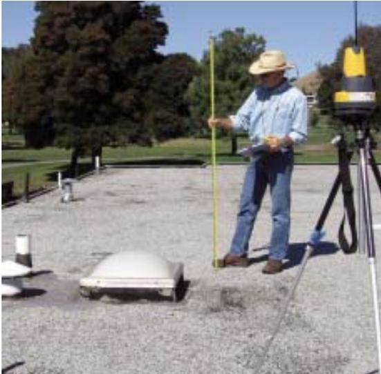
**Figure 1.** The author uses a laser level to measure the elevation at various points on the roof (above) and then records the information (right). The map tells the applicator where the low spots are so he can build up those areas with a thicker layer of foam and thereby prevent ponding.
