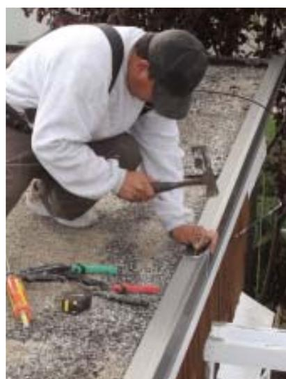
**Figure 3.** Before SPF is applied, the existing gravel stop is removed (above) and replaced with a new stop designed for foam. The crew uses polyurethane sealant and at least two nails at every lap (right) to prevent the joints from flexing and cracking. Next, the stop is nailed 9 inches o.c. to the edge of the roof.
